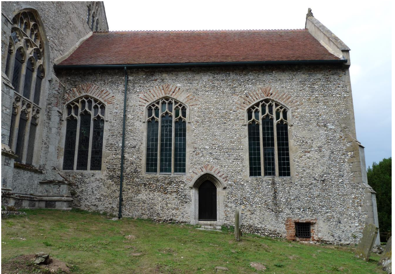
Fig.2 Note how the chancel windows are crowded towards the west (left hand) end
